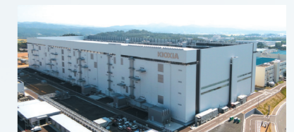
Kitakami Plant of Kioxia Iwate Corporation
