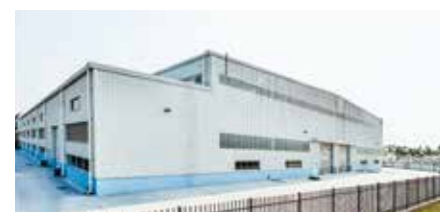
External view of new casting plant
