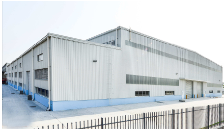
External view of new casting plant
