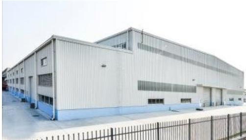
External view of new casting plant
