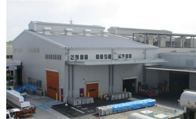
Plant No. 6 exterior
