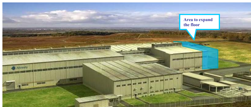
Image of the area to expand the floor of the casting plant in Ahresty Mexicana
