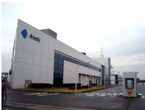
Exterior of Head Office/Technical Center
