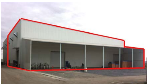
Expanded area at the die casting plant
