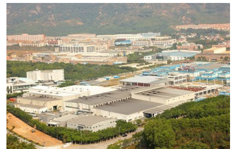
First Plant and New Plant (as of January 2013)
