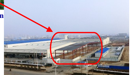
Scene of third-phase construction (Processing plant/storehouse)
