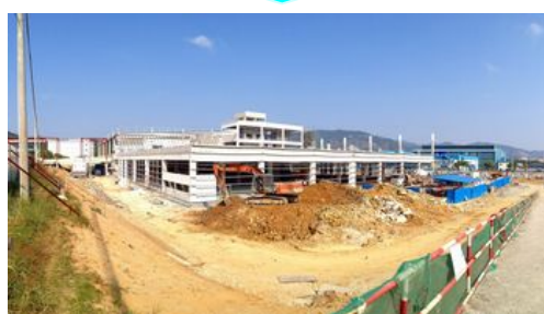
Scene of new plant construction (as of January 2013)
