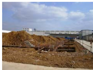
Processing plant under construction at Hefei Ahresty
