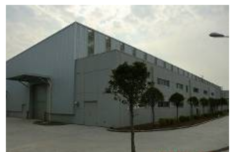
Second expansion completed at Ahresty Precision Die Mold (Guangzhou)
