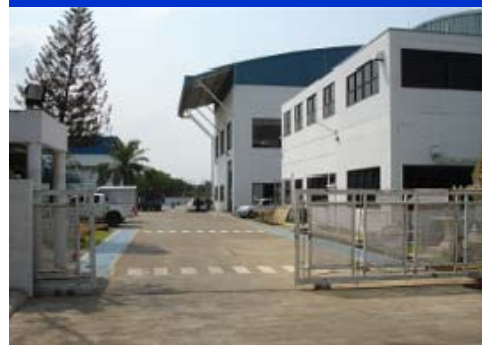
Feb. 10, 2012 Reconstruction almost complete
