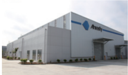
New plant of Ahresty Precision Die Mold (Guangzhou) Co., Ltd., construction of which has been completed
